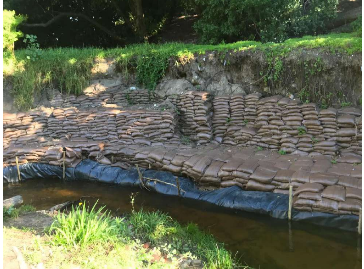
Temporary erosion control on Hout Bay Common
